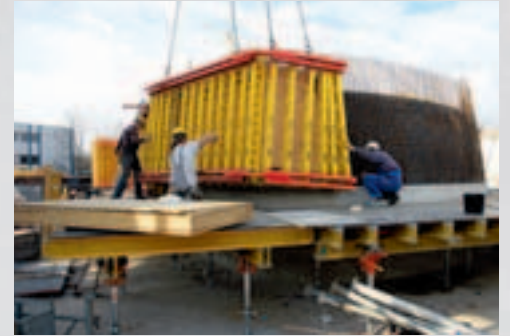
Assembly on the construction site
