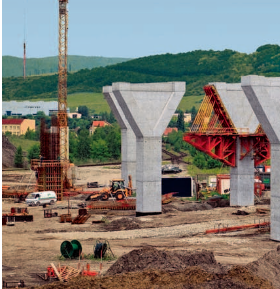
For constructing the pier heads, PERI's team of Czech engineers developed an efficient formwork solution with horizontally-positioned SB brace frames and VARIO GT 24 girder wall formwork.
