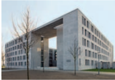
A massive reinforced concrete roof over the entrance to the inner court harmoniously closes the connection of the individual building sections.
