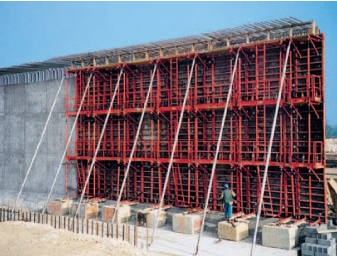
Extended TRIO panels for 8.00 m high walls.
