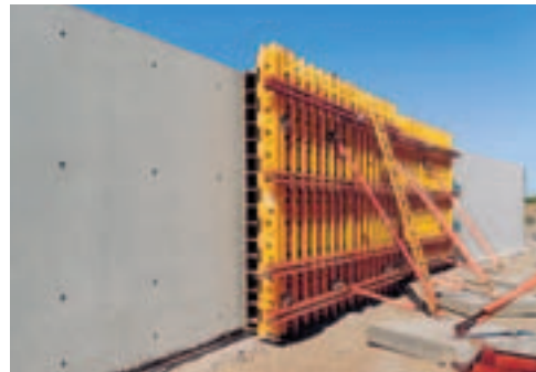
Excellent architectural concrete result thanks to the VKS coupling for architectural concrete.
