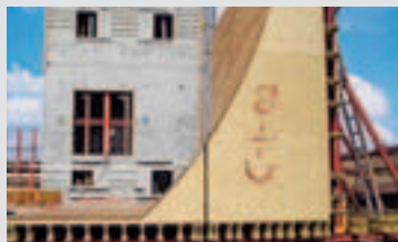
Use of complete formwork elements on the construction site.
