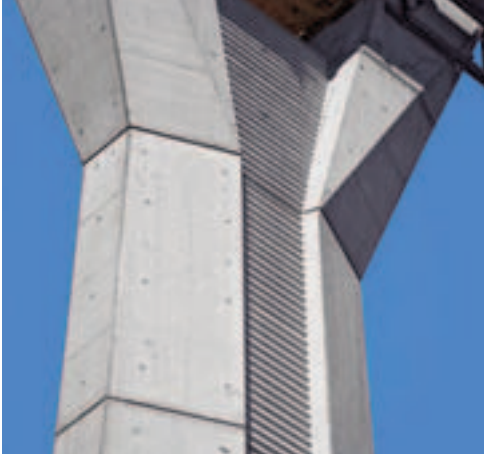
Viaduct Schleuse, Schleusingen, Germany
