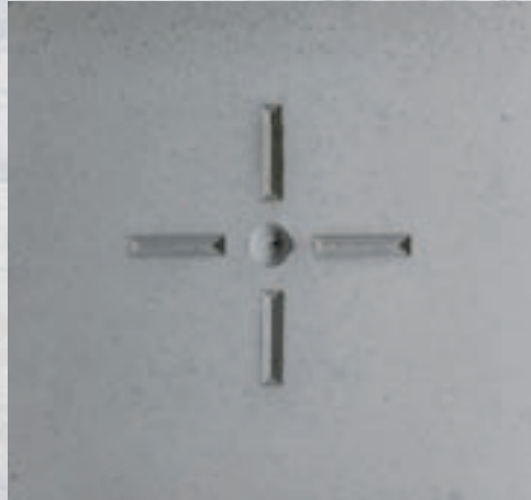
Tie point plugged with blind anchor
