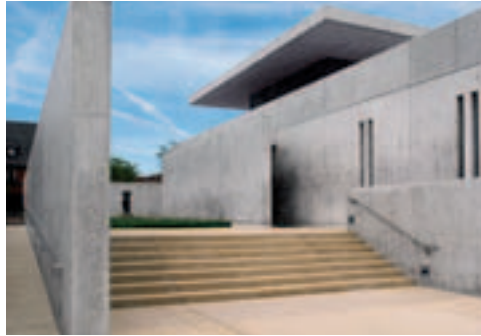
The Pulitzer Foundation for the Arts is an impressive architectural concrete building designed by the Japanese architect Tadao Ando and realised using PERI formwork technology.
