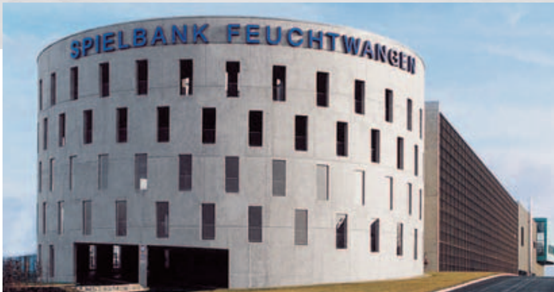
Architectural concrete facade of spiral ramp with a neat joint arrangement.
