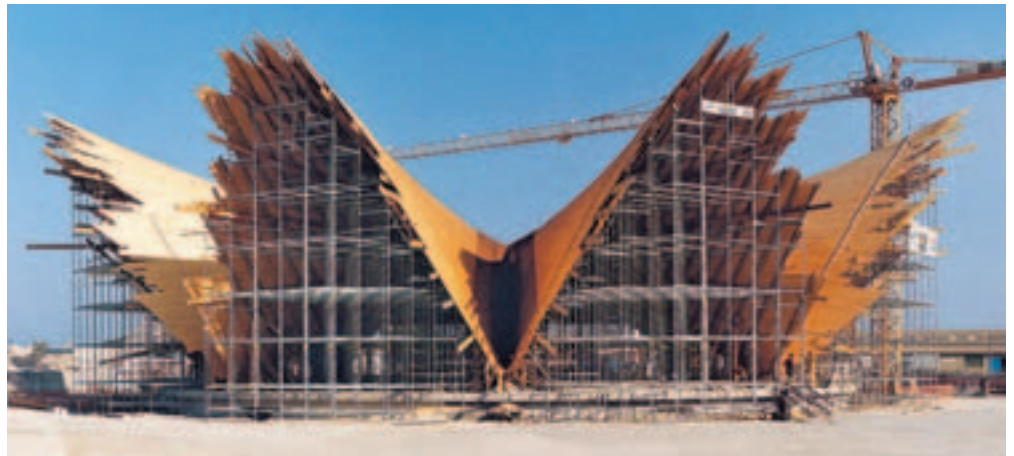
The PERI Rosett falsework reached a height of 13.70 m.
