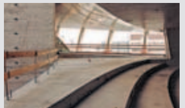
The result: sharp edges, highest quality surface finishes and a uniform tie arrangement.
