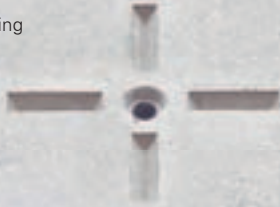
Tie point plugged with blind anchor
