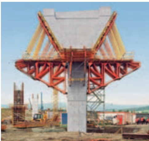
For constructing the pier heads, PERI's team of Czech engineers developed an efficient formwork solution with horizontally-positioned SB brace frames and VARIO GT 24 girder wall formwork.
