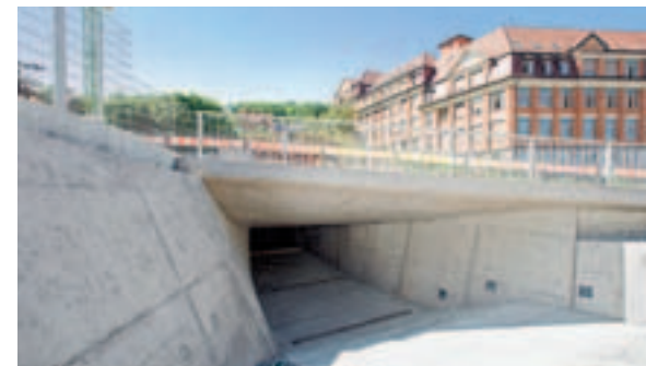
Successful result: accurately executed forms with a high surface quality. The pre-assembled 3D formwork from PERI is joined together and positioned with millimetre precision on the construction site.
