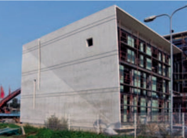
The result speaks for itself. Due to the excellent teamwork between architect, contractor and formwork supplier, first-class results were achieved.
