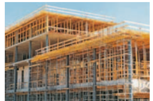
Girder slab formwork MULTIFLEX
