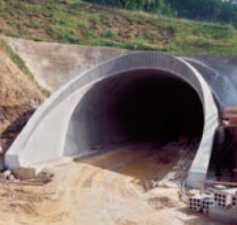
Sommerberg Tunnel, Hausach, Germany
