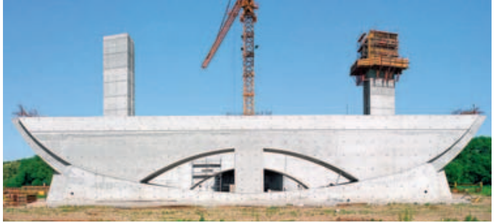
... resulting in a very accurate construction as well as in the required surface quality.
