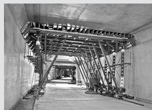
Tunnel formwork
