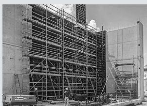
Working scaffolds for construction
