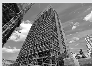
Working scaffolds for facades
