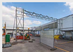
Scaffold bridges for power cables
