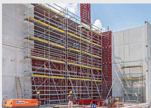
Working scaffolds for construction
