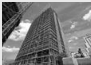
Facade working scaffold
