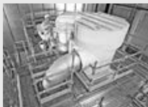
Working scaffolds industry
