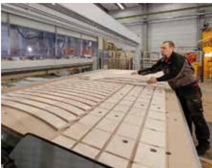
Using state-of-the-art CNC machines, panels are cut ensuring the highest precision and completely in accordance with the specifications of the PERI CAD plan file.
