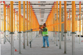
Slab Formwork
