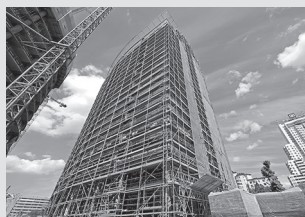
Working scaffolds facade
