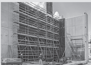
Working scaffolds construction
