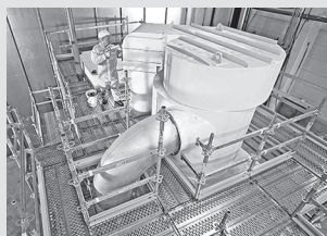
Working scaffolds industry
