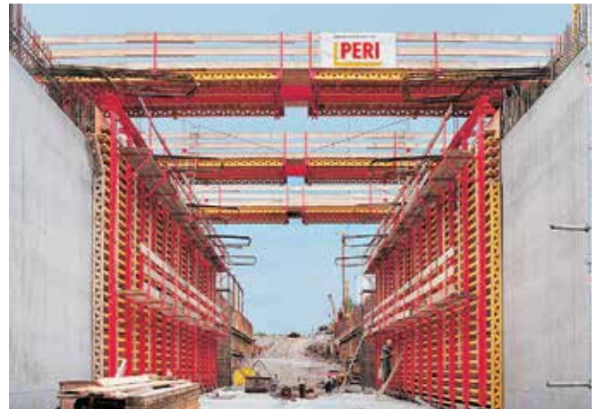
B311 Local Bypass Tunnel, Ertingen, Germany.
