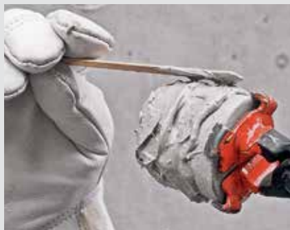
Hold the concrete cone with a pair of cone pliers, and coat its tapered surface and end evenly with sealing compound.
