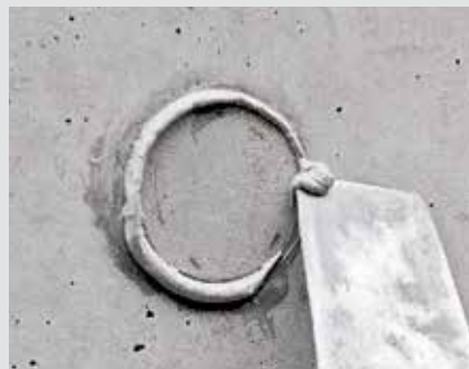
Scrap the surplus compound off with a filling knife.
