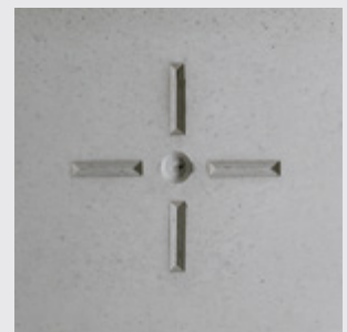
Formwork panel with blind cone
