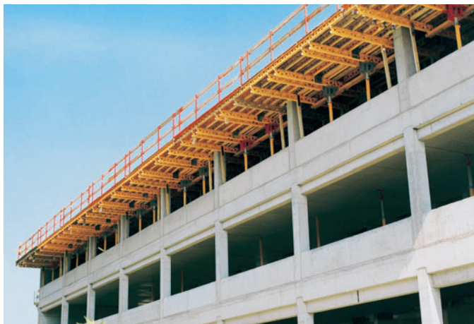
Cantilevered PERI UNIportal edge tables with guardrails.
