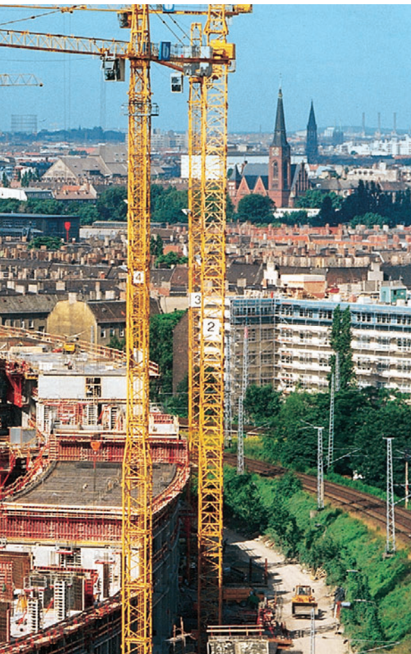
UNIportal slab tables for constructing an administration building.
