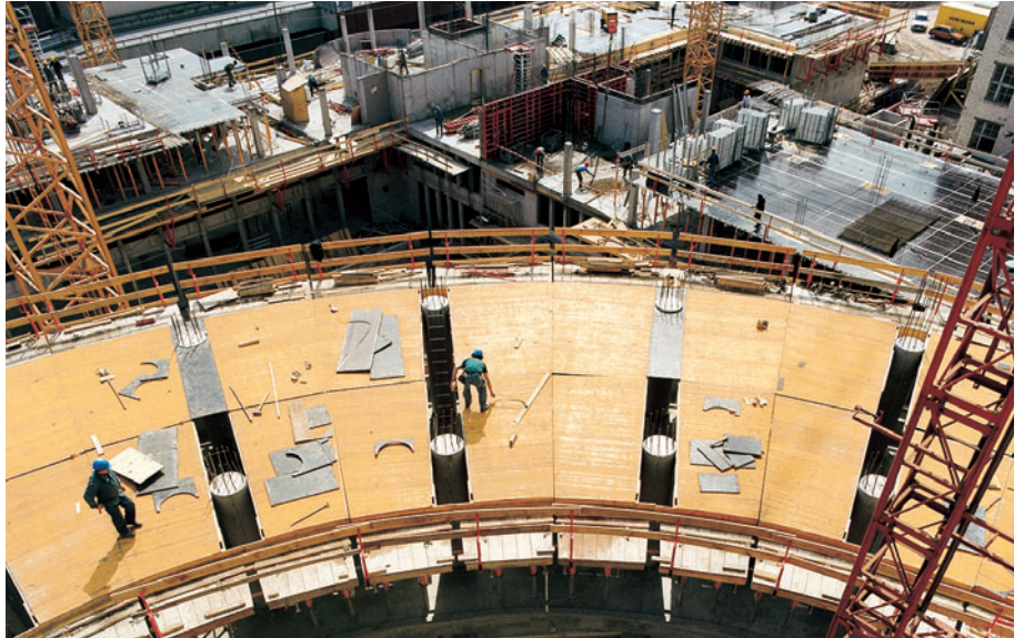
The fillers are located at the column areas.
