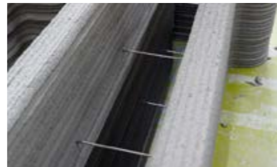
The BOD2 is the fastest machine of its kind on the market. It takes only about five minutes to produce 1 m 2 of cavity wall.
