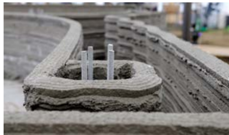
It is already possible to obtain BOD construction permits for buildings by integrating reinforcement and filling the hollow spaces.
