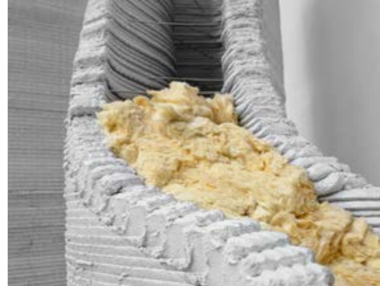
The insulation can be integrated into the printed, double-shell cavity walls.
