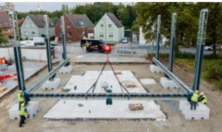
The BOD2 is suitable for producing the walls of your project. Foundations and ceilings are constructed in a traditional manner.
