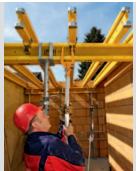
Using the same Fixing Tool, the Flexclips are also safely mounted from the ground.
