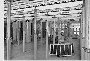
Slab Formwork
