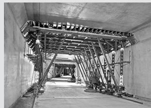
Tunnel Formwork
