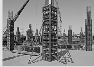
Column Formwork
