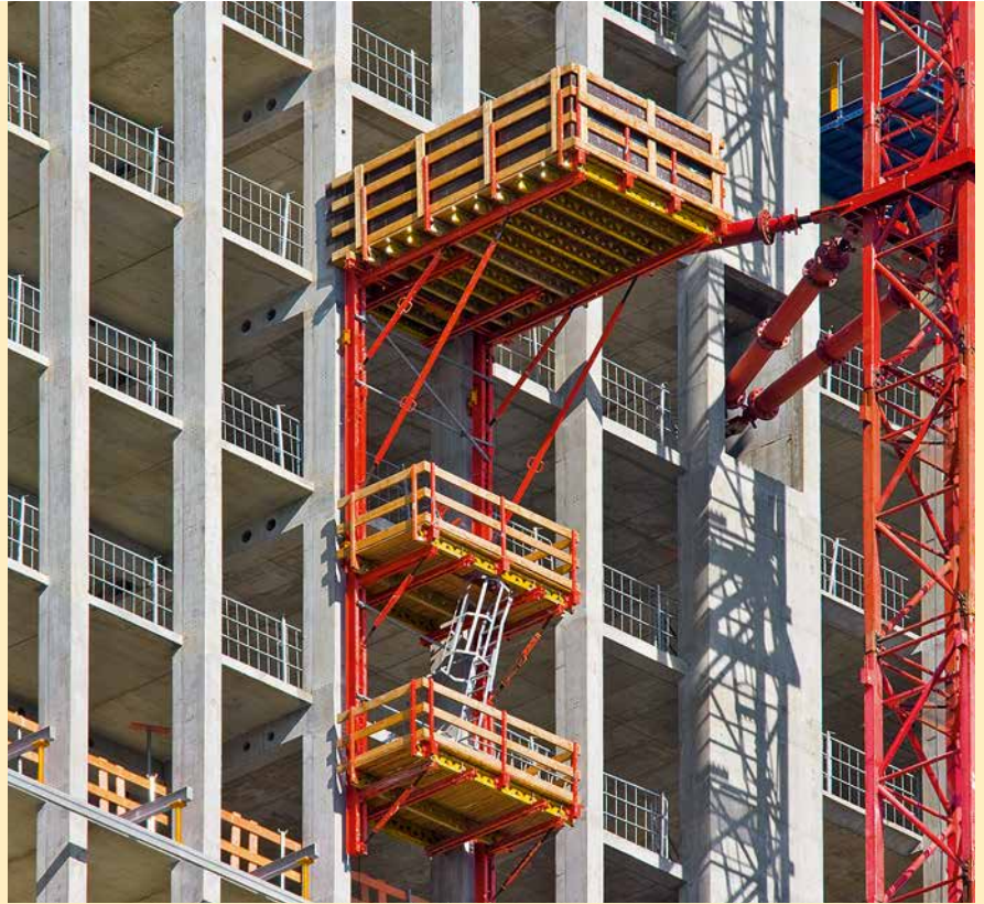
This self-climbing RCS Bracket Platform with 2 finishing platforms on a high-rise building is anchored in the facade columns by means of the RCS Wall Shoe.
