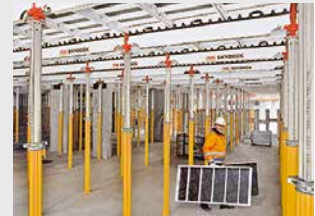
Slab Formwork
