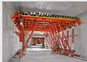
Tunnel Formwork
