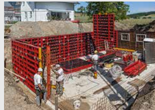
Wall Formwork
