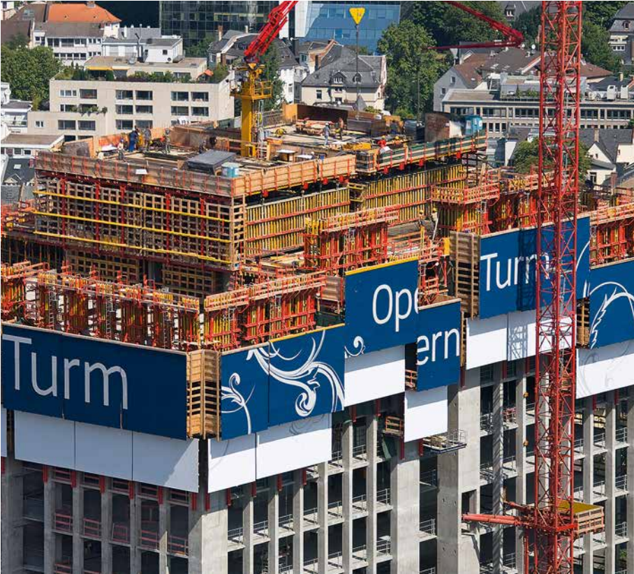
RCS provides safe working areas at the highest level – here completely enclosed.
