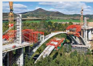
Bridge Formwork
