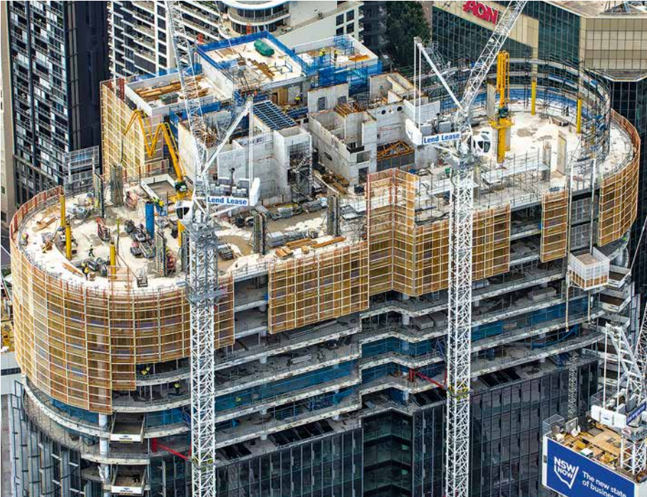
In Australia, mesh enclosures are frequently used due to the high temperatures. This allows not only air but also light to enter the building.
