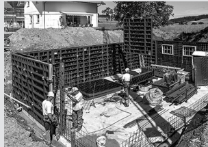
Wall Formwork
