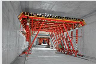
Tunnel Formwork
