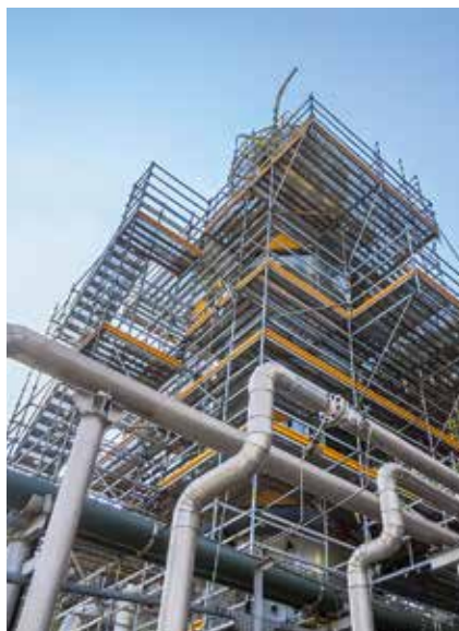
Stair towers with staircase units in the same direction have the advantage that, in addition to staircase units, working levels are also available.
