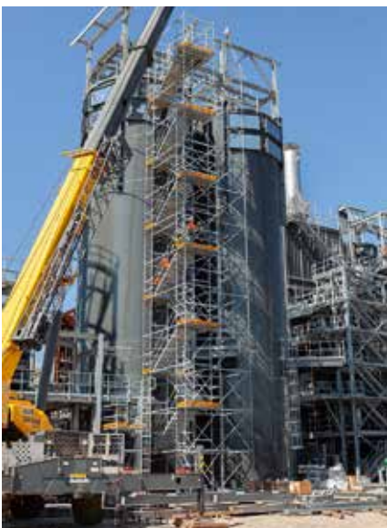
Stair towers with alternating staircase units provide greater head clearance and shorter walking distances for site personnel between levels.
