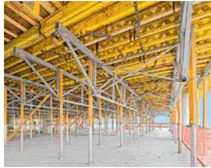
MULTIPROP Props, used for large-sized SKYTABLE Slab Tables, facilitate faster cycles with a higher level of safety.
