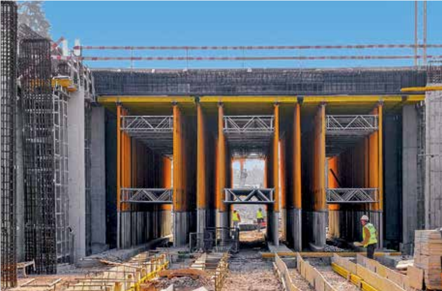
Especially with large slab heights, MULTIPROP Shoring Towers are a cost-effective alternative to standard spatial load-bearing scaffold.
