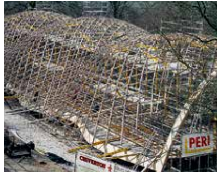
MULTIPROP Props carried the timber construction and facilitated the curved shape of the gridshell.
