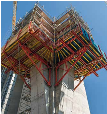
Horizontally mounted Brace Frame system combined with system components of the VARIOKIT Engineering Construction Kit form cantilevered working platforms.
