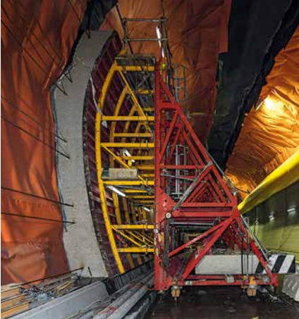
For single-sided concreting, the Brace Frame transfers the high loads into the foundations.
