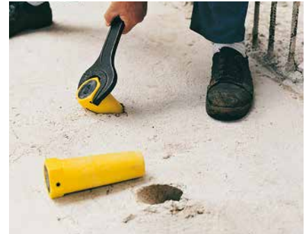
The Leading Anchor Coupler can be recovered after concreting.
