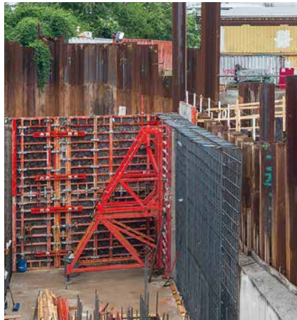
When concreting single-sided against existing sheet piling, the entire fresh concrete pressure is transferred into the sub-structure via the Brace Frame complete with corresponding anchorage.
