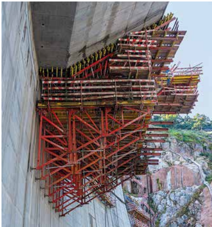
Brace Frames and system components taken from the VARIOKIT Engineering Construction Kit form large-sized platforms up to 8.75 m wide.
