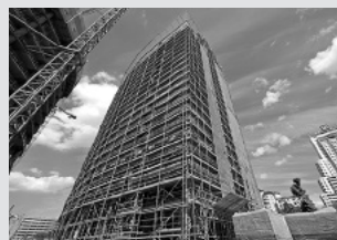
Working scaffolds for facades
