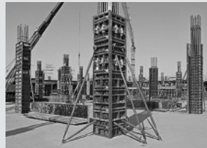
Column formwork
