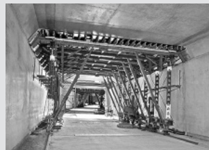
Tunnel formwork
