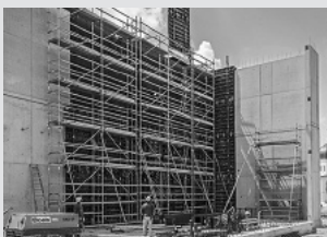
Working scaffolds for construction
