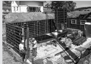
Wall formwork
