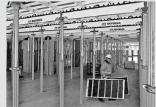
Slab formwork
