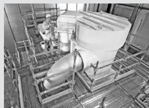
Working scaffolds for industry
