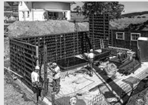
Wall Formwork
