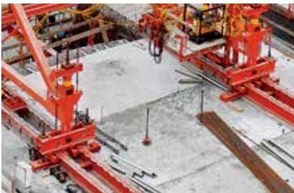
Lower workload Only 2 anchors per A-frame required.
