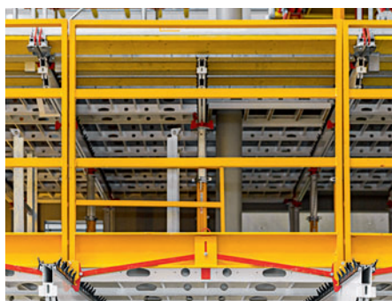
Guardrail unit with a width of 150 cm in use.
