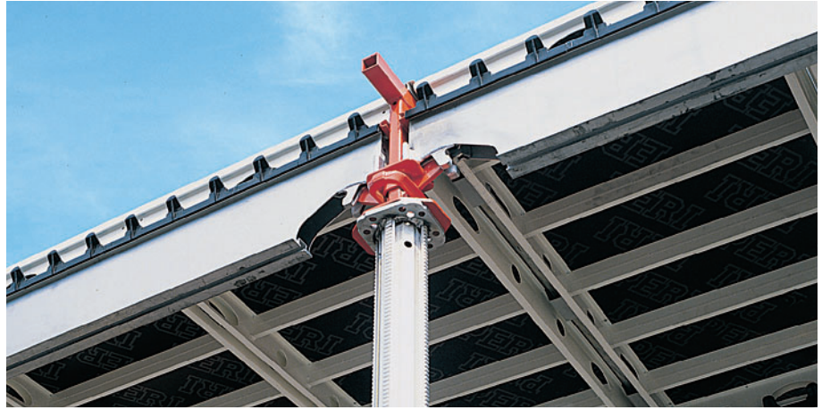
The drophead system in the SKYDECK standard field.
