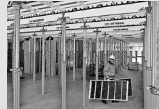
Slab Formwork
