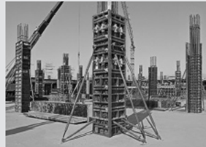
Column Formwork
