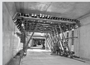
Tunnel Formwork
