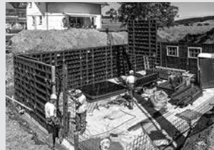
Wall Formwork
