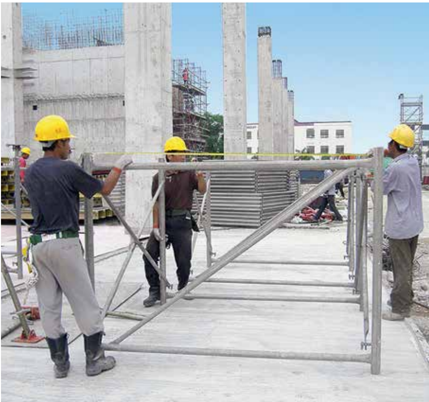
Basic assembly of the PD 8 Shoring can be carried out manually.
