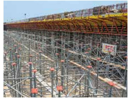
The high load-bearing capacity of the PD 8 System in connection with steel walers as main beams facilitated cost-effective working.
