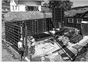
Wall Formwork
