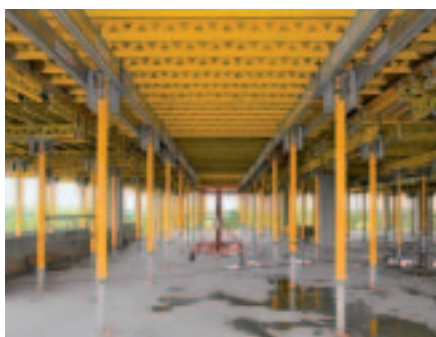
The MPB 24 beam used as a dou- ble main beam for slab tables.
