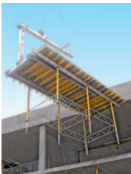
With the PERI transportation fork, tables up to 8.0 m long and weigh- ing 1.75 t can be moved.
