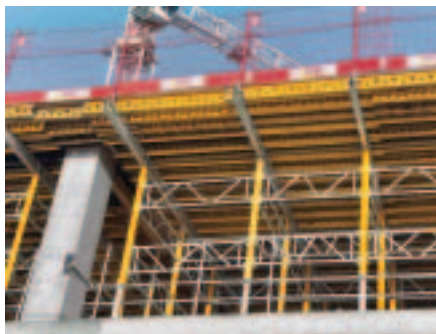
The MULTIPROP frame provides the required stability for the edge tables.
