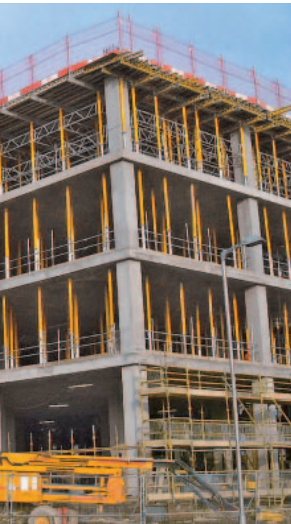
An ideal combination: MULTIPROP props with frames, MPB 24 beams as main beams and GT 24 as cross beams.
