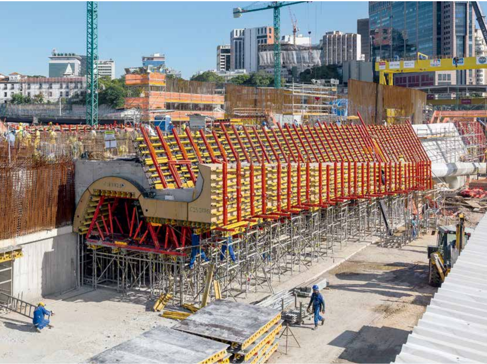
Supported by PERI UP shoring and working scaffolds, as well as a VARIOKIT raised formwork unit, the customised elements could be assembled on-site to form a complete 3D formwork construction.
