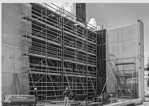
Working scaffolds construction
