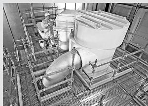
Working scaffolds industry
