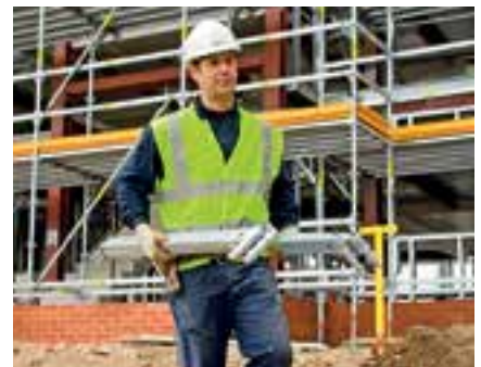
The small width of the UH Ledger allows up to 4 ledgers to be carried at any one time by one scaffolder.
